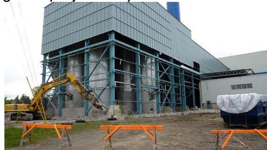
Exterior demolition of the coating kitchen building in preparation for the removal of the tanks.
